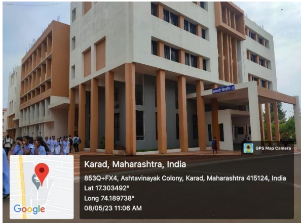
Shatabdi Building- E
